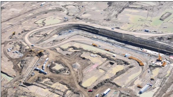
Above: Storm pipe installation at Taxiway Juliet
