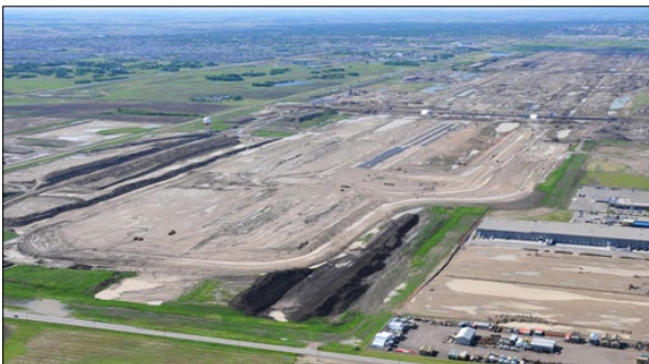
Above: Runway Grading -View from the North
